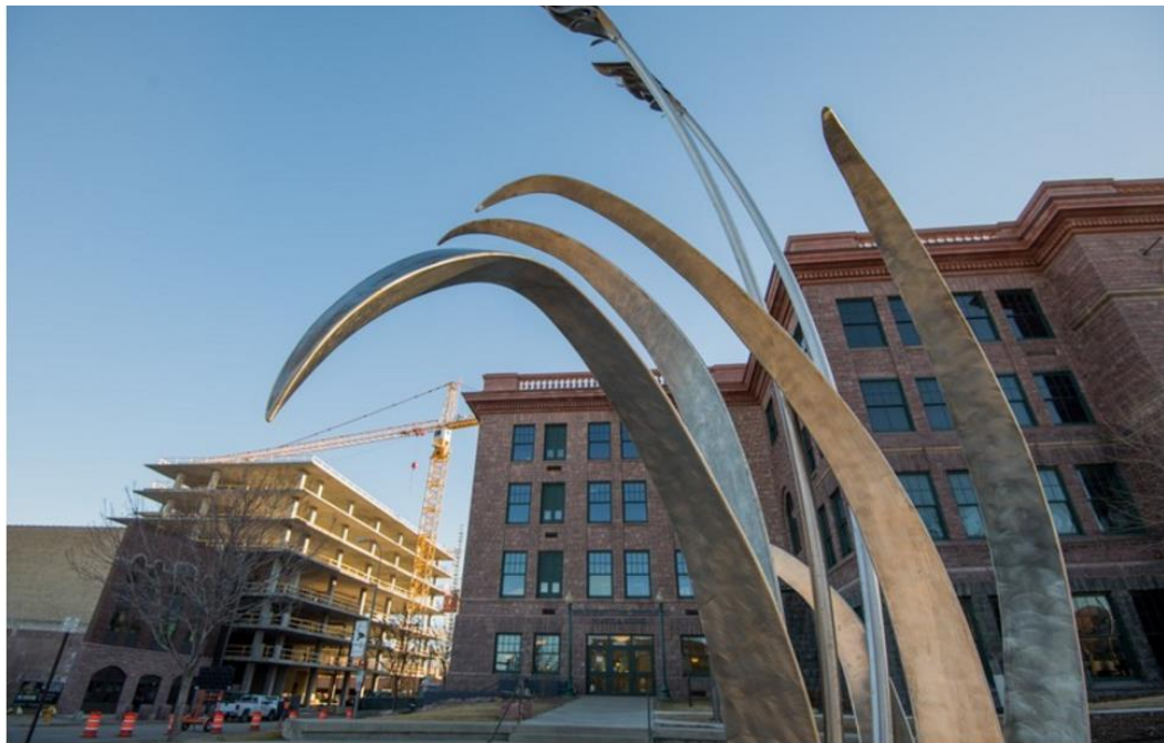
Construction continues on the Washington Square building next to the Washington Pavilion in downtown Sioux Falls earlier this month.
